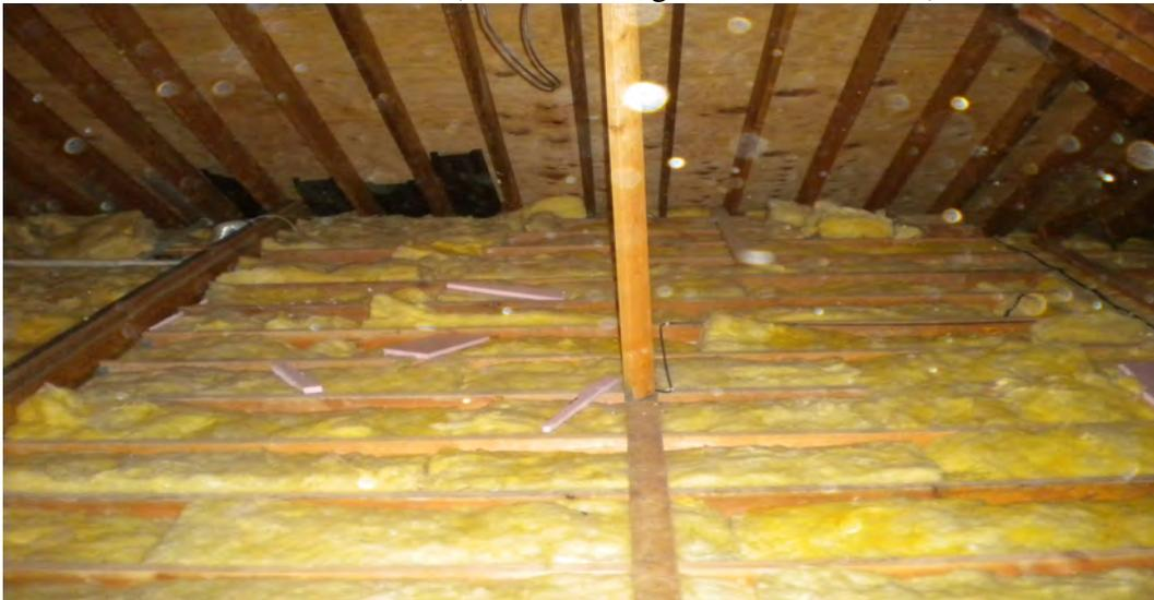
After additional insulation (8 inch fiberglass batt insulation with 8+ inches of blown cellulose insulation) R-Value 49
